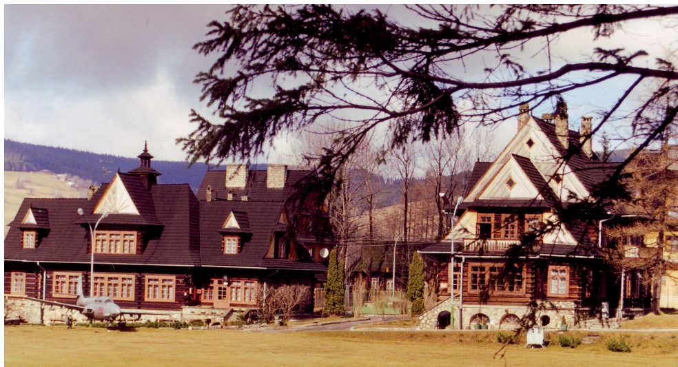
III. 4. A complex of wooden buildings designed by Stefan Mejer, Kościelisko – Gronik
