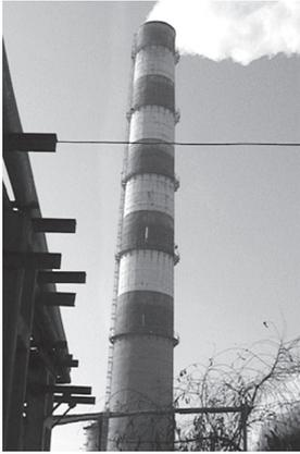
Ill. 5. Iron concrete monolithic pipe  $H = 120$  m
