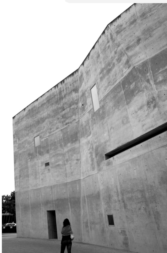
III. 26. Freiburg, St Maria Magdalena's Church, designed by Kister Scheithauer Gross Architekten, 2004
