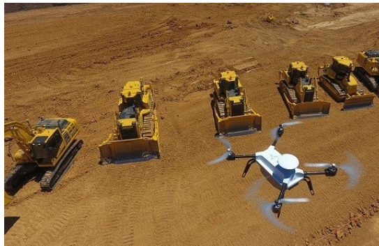
Fig. 1. Quadcopter assisting in construction works (source: komatsu.com)
