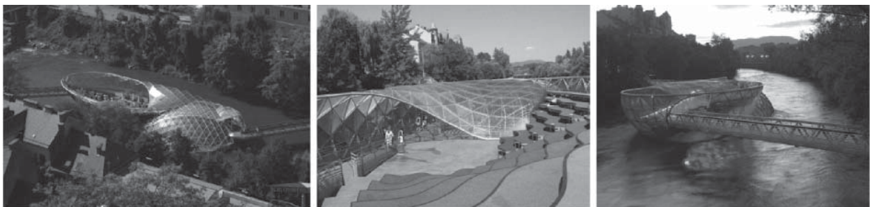
il. 7. Mur Island Bridge, Graz, Austria, 2003 by Acconci Studio (Photos by Acconci Studio).
