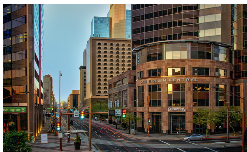
Fig. 23. Phoenix, Arizona, modern urban fabric downtown, source; High Street AZ, http://www.highstreetaz.com
