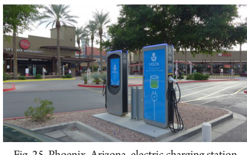
Fig. 25. Phoenix, Arizona, electric charging station inside a retail center in Phoenix, source: Inside EVE, https://insideevs.com/volta-industries-approaching-500-charging-station-across-the-us/
