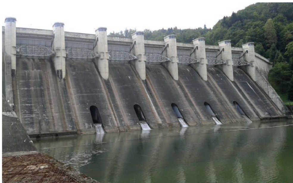
Fig. 1. Rożnów Dam [source: author's own]
