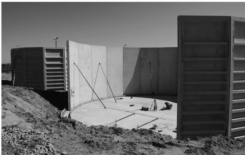
Fig. 2. Tank erection
