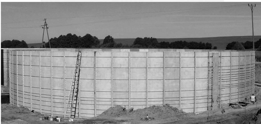
Fig. 1. Circular tank made of precast components
