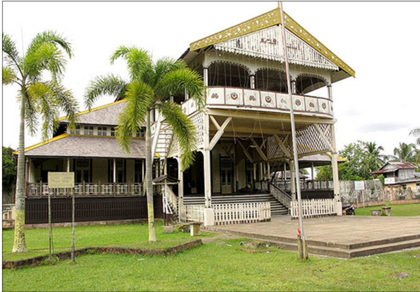
Fig. 2.4a. Istana Kadariah Pontianak with kolong at ground level, verandah at upper level and mass tiered roof to the entire length of building that facilitate wind driven ventilation and maximum turfed ground surface prevent buildup of heat island and surface water runoff. (Source: flicker images)
