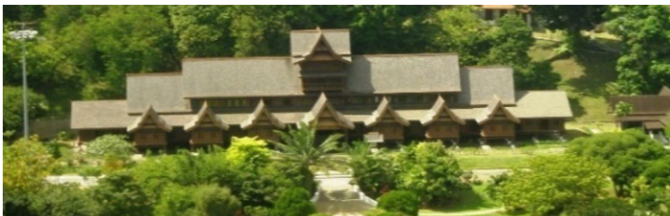
Fig. 2.1a. The essentially elongated massing of the palace is suited to enhance wind driven ventilation which can be of horizontally and vertically facilitate through the Melaka palace vernacular form. linear building, mass tiered roof form and the kolong – floor underspace
