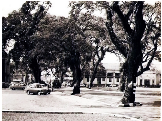
Fig. 2.5a. Original tree lined street in Alor Setar, in front of the royal palace
