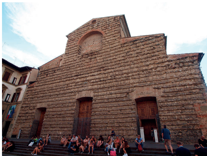
III. 4. Firenze, technical fraying of the unfinished main elevation of the San Lorenzo basilica (photo by author)
