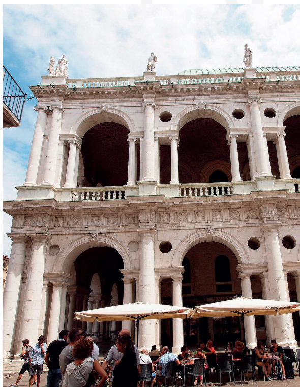
Ill. 9. Vicenza, architectural composition of loggia, so-called palladian motive of the basilica (photo by author)
