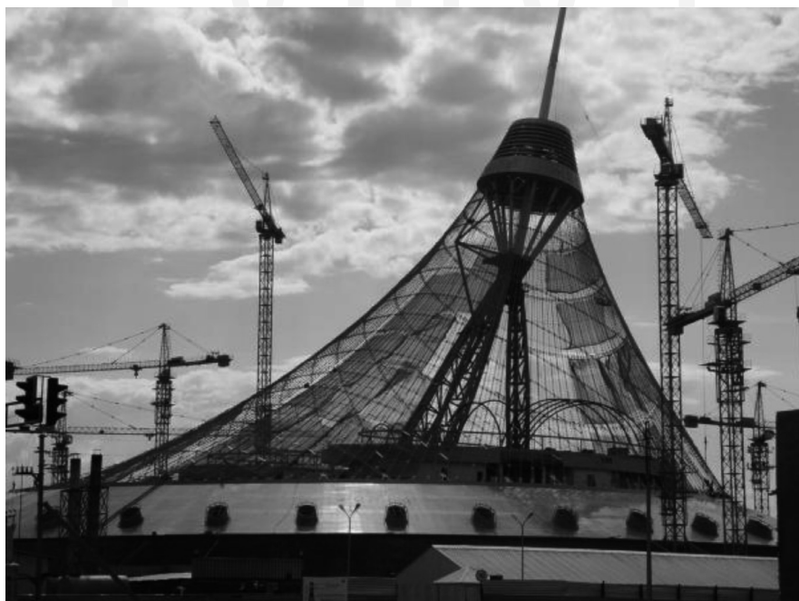
III. 3. A general view of the “Khan Shatyr” during the construction period (source: Conceptual design of Khan Shatyr, Foster and Partners)
