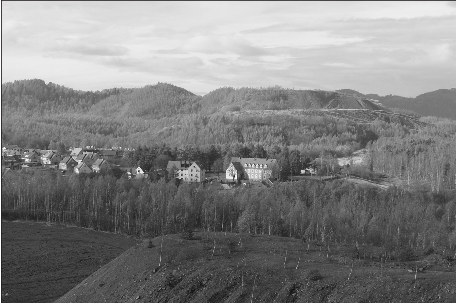
Photo 1. Anthropogenic inversion of relief in the Wałbrzych coal mining area. Landscape of the largest dump of the Wałbrzych coal mining area (50.0 hectares, 23.077 mln m 3 , 105 m), (photo by J. Wójcik)
