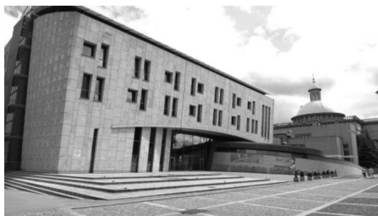
Ill. 1. Faculty of Theology, University of Silesia in Katowice (2004). Entrance facade (photo D. Winnicka-Jasłowska, 2013)
