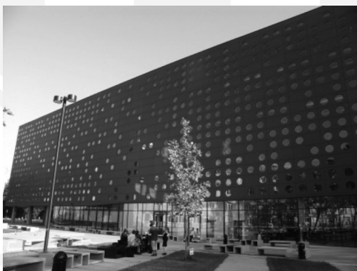
III. 3. Integrated Student Centre at Wrocław University of Technology (C-13) in Wrocław (2007) (photo D. Winnicka-Jasłowska, 2013)
