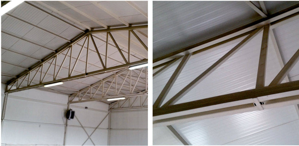
Fig. 1. Lattice girders made from closed and open steel sections
