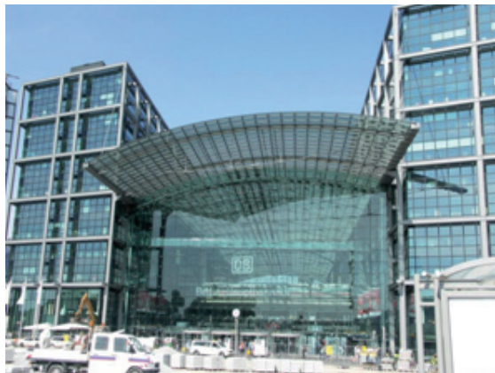
Ill. 33. Central Railway Station (Hauptbahnhof/Lerther Bahnhof) – southeastern entrance (photo by Z. Zuziak)
