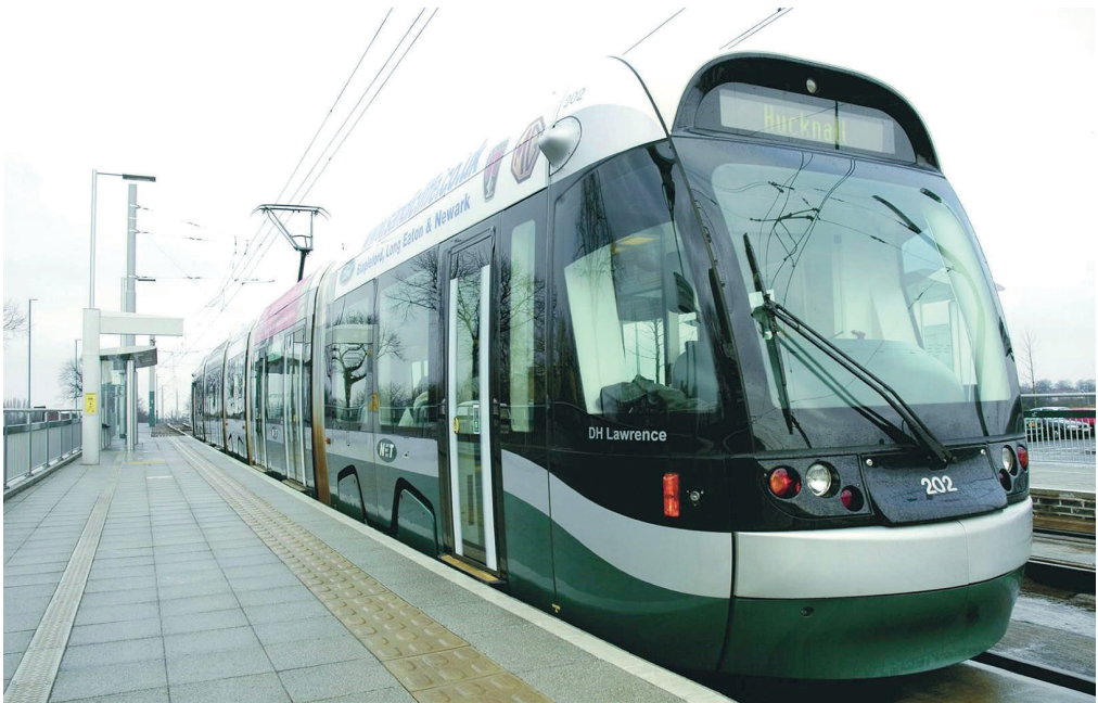
Fig. 4. Platform edge warning surface on a tram stop (source: www.marshalls.co.uk , accessed 10.03.2018)
