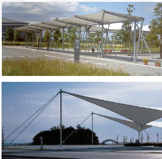
Fig. 1. Free-standing canopy roofs of membrane structures, a) mono-sloped, b) HP-shaped
