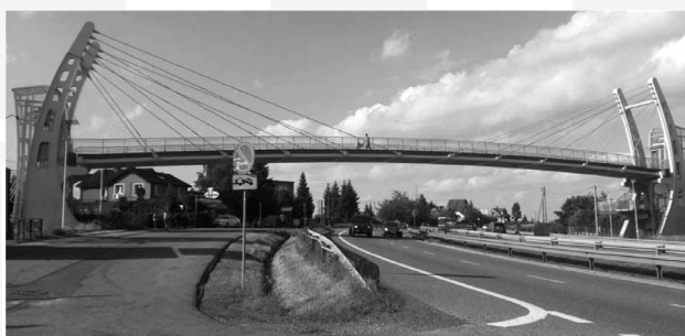
Fig. 2. The footbridge over the S7 national road 'Zakopianka' located in Gaj
