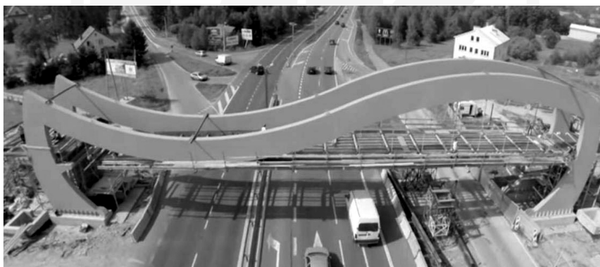
Fig. 4. The footbridge located in Jawornik
