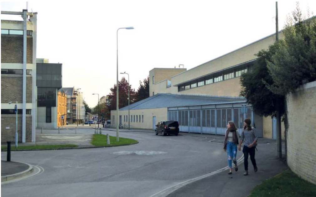
Fig. 16. A side elevation with only service doors facing the street (photo by I. Samuels)
