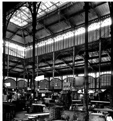
III. 5. Paris, Les Halles – the interior; designed by V. Baltard and F. Callet (1853–1870) (source: http://rubens.anu.edu.au/ htdocs/laserdisk/0231/23127.JPG )
