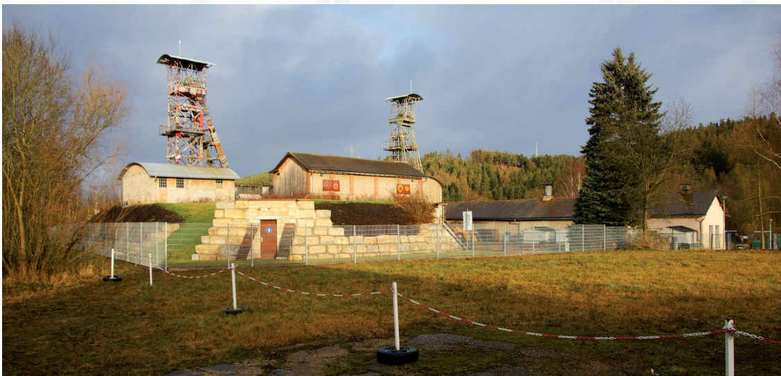
III. 6. Shaft building complex of iron ore mine “Maffei” in Auerbach-Nitzlbuch, with specific headframes (photo by author, 2013)
