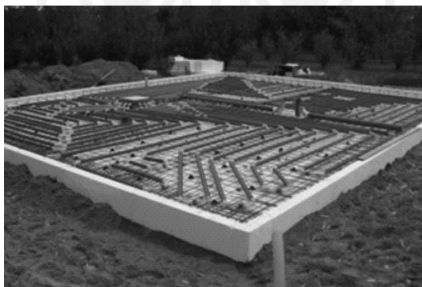
Fig. 1. The exemplary heating foundation [5]
