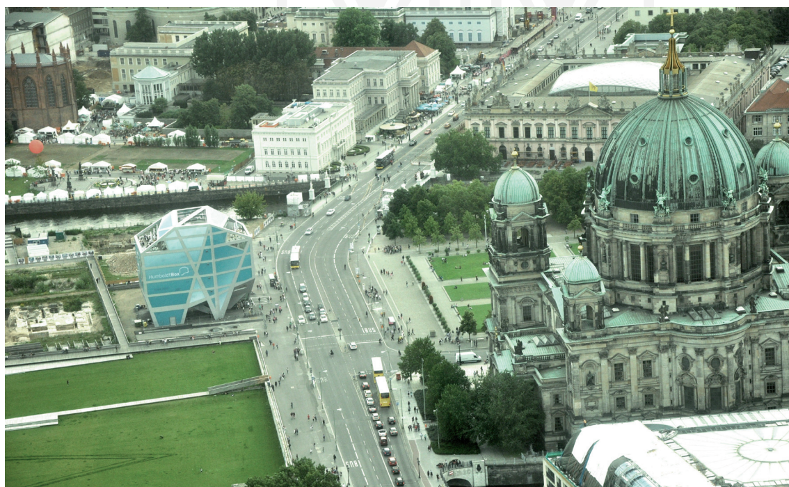
III. 2. Context of the planned reconstruction of the historical Berlin Castle and the GDR Palace demolished in 2008, temporary blue “Humboldtforum” nearby (photo by K. Racoń-Leja)
