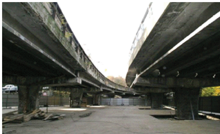
Fig. 2. View of viaduct before repair
