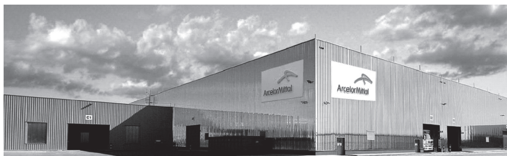
Fig. 6. Stainless steel façade of ArcelorMittal – Stainless Service Poland Sp. z o. o. building in Siemianowice Śląskie, Poland [2]
