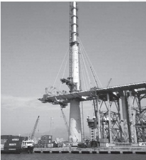
Fig. 2. Structural use of stainless steel in road bridges: towers of Stonecutters Bridge, Hong Kong, China [1]
