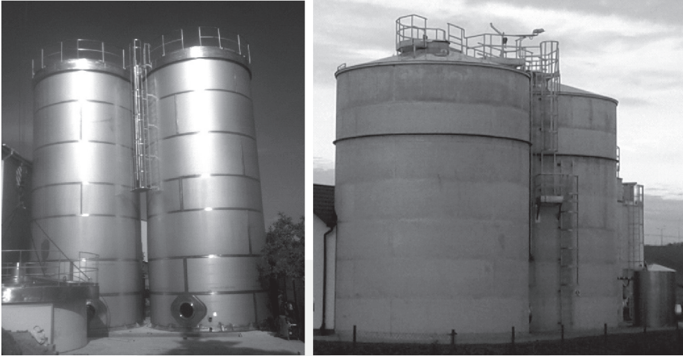
Fig. 7. Example of structural use of stainless steel in Poland – tanks (305 m 3 ) for concentrated fruit juice, Spomasz Zamość S.A., Poland, A. Biczak – author of photography (left) and tanks (490 m 3 ) in sewage-treatment plant in Targowisko, municipality Klaj, Poland, P. Żwirek – author of photography (right)
