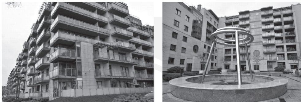
Fig. 9. Apartment complex “Wiślane Tarasy”, Cracow, Poland (contractor: INTER-BUD, structural stainless steel elements design: K. Kuchta, P. Marzec, I. Tylek)
