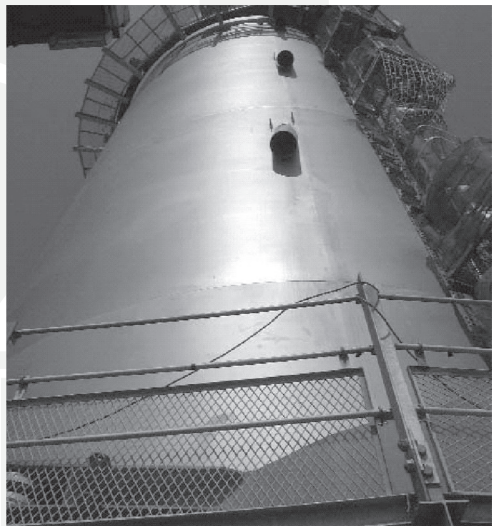
Fig. 2. Structural use of stainless steel in road bridges: towers of Stonecutters Bridge, Hong Kong, China [1]
