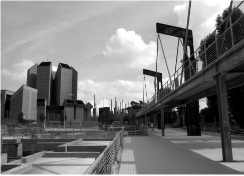
Fig. 16. The Church of Santo Volto is visible from the side of post-industrial areas revitalised for recreational purposes. On the right, there is a footbridge connecting the areas of former factories (photo by: M. Jagiello, 2013)
