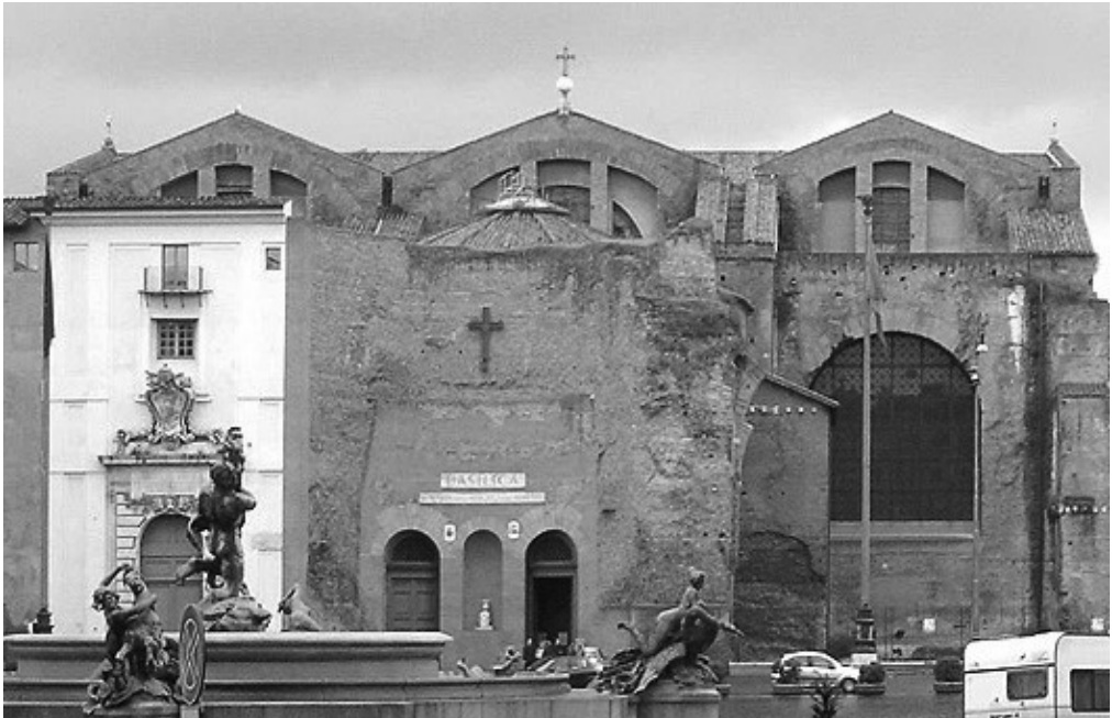
Fig. 2. Entrance to the Basilica of Maria degli Angeli e dei Martiri, created on the site of the former Diocletian bathing complex and adapted for the sacred function following the design of Michelangelo, around 1598 (photo by R.A. Frantz, 2005; source: [25])
