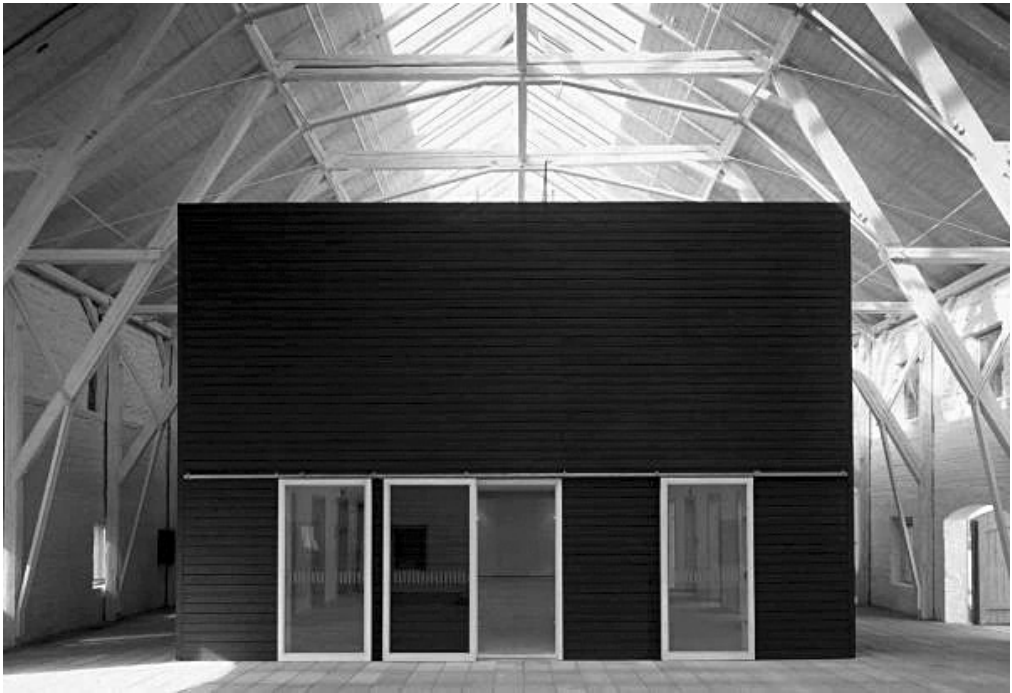
Fig. 10. The parish house in the former barn (building within a building) of the parish complex in Schwindkirchen (source: [29])
