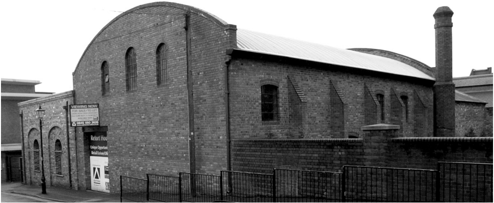
Fig. 12. View of gas buildings with their characteristic chimney, after maintenance, with the main entrance to the present church (source: [31])
