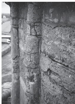
Fig. 6. a) damage of prefabricated shell elements four years after repair; b) exhaust chimney near the tower
