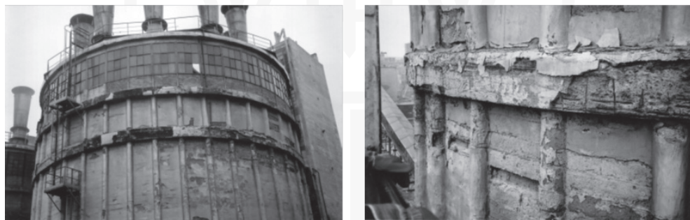
Fig. 4. Corrosion of the prefabricated cylindrical shell (2002)
