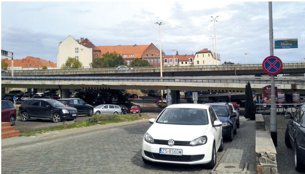
Fig. 7. Szczecin – a grade-separated junction of Nadodrzańska Artery (built right after World War II) and Zamkowa Route generates nobody's land in the very city centre, which dangerously hampers the creation of any compositional and functional link between both parts of the Old Town (photo by K. Dudzic-Gyurkovich)
