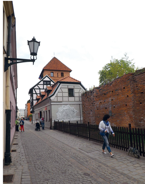
Fig. 4.b. The name and course of Podmurna street ( Polish: near the walls ) in Toruń testifies to the presence of fortifications whose fragments have been preserved to date (photo by K. Dudzic-Gyurkovich)
