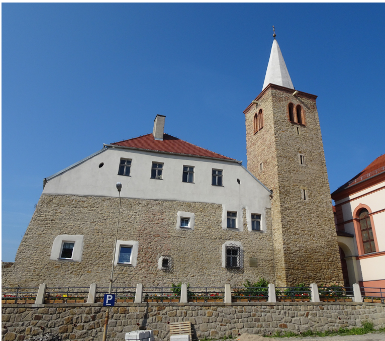
Fig. 4. a) Bystrzyca Kłodzka, Rycerska (Knight's) Tower, view from the south (before conservation works) (photo by A. Legendziewicz), b) Bystrzyca Kłodzka, Rycerska (Knight's) Tower, view from the north (after conservation works) (photo by A. Marcinów)
