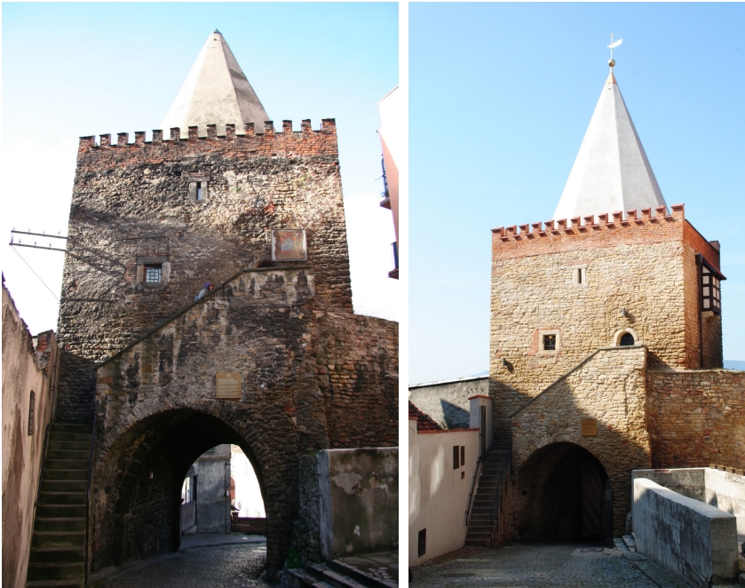
Fig. 3. a) Bystrzyca Kłodzka, Wodna (Water) Gate, view from the north (before conservation works) (photo by A. Legendziewicz), b) Bystrzyca Kłodzka, Wodna (Water) Gate, view from the north (after conservation works) (photo by A. Marcinów)
