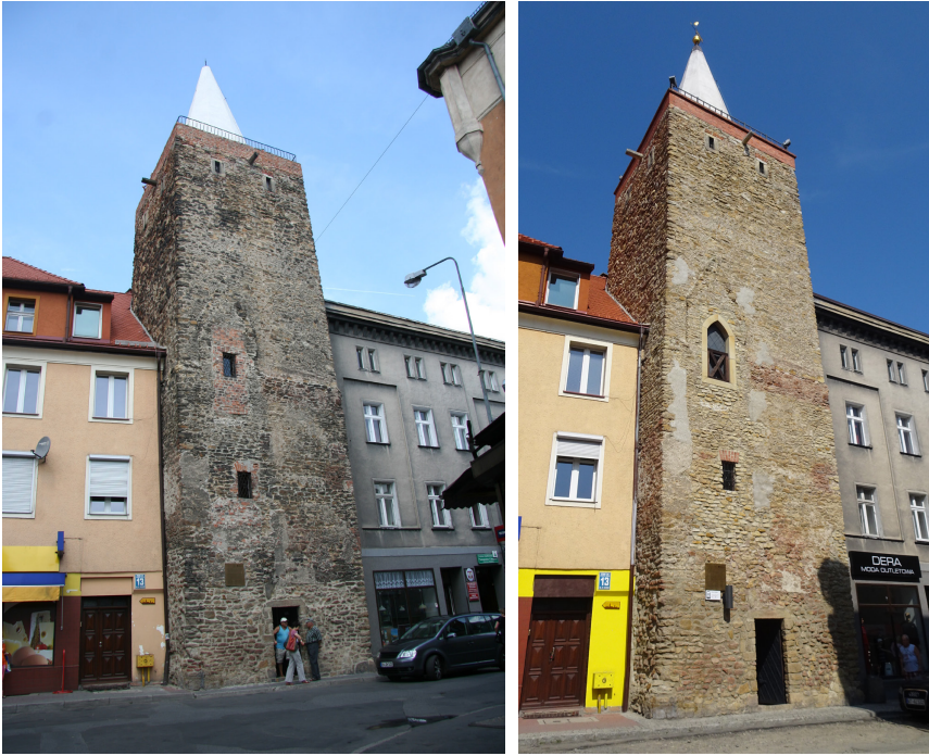
Fig. 1. a) Bystrzyca Kłodzka, Kłodzka Gate's tower, view from the east (before conservation works) (photo by A. Legendziewicz), b) Bystrzyca Kłodzka, Kłodzka Gate's tower, view from the east (after conservation works)(photo by A. Marcinów)
