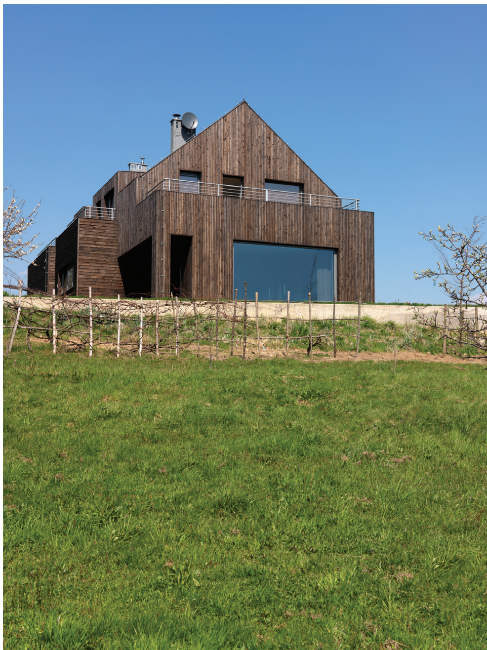
III. 3. House in Burów, view from the south, photo Wojciech Kryński, courtesy of Stanisław Deńko and the office 'Wizja' sp. z o.o.
