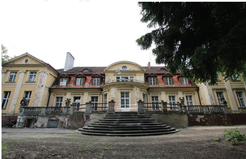
III. 2. Pałace in Bieganowo, garden elevation with a terrace, current condition (photo by J. Białkiewicz)
