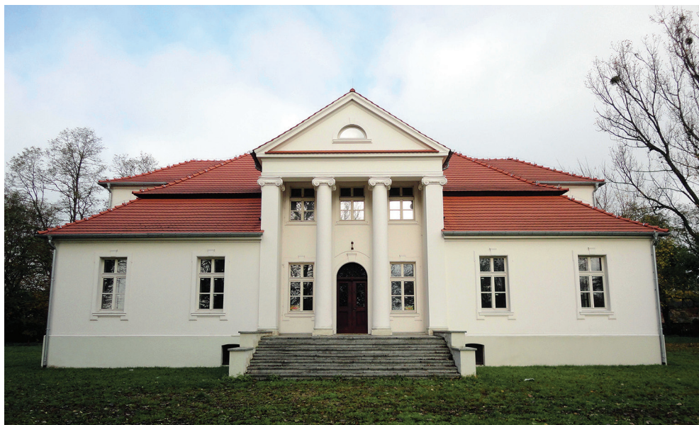
III. 3. Mansion in Wódki, front elevation, current condition (photo by J. Białkiewicz)
