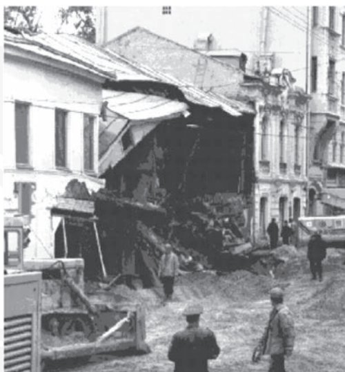
Fig. 4. A building destroyed due to ground uplift from under the foundation to a tunnel executed below, Moscow 1998 [15]
