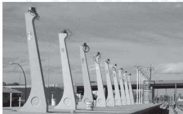
III. 7. Application of RPC (Reactive Powder Concrete) – “Ductal®”: Shawnessy Light Rail Train (LRT) Station (RPC precast elements: ultra-thin (2 cm) curved roof shell, columns), Calgary, Canada, 2004 [40]
