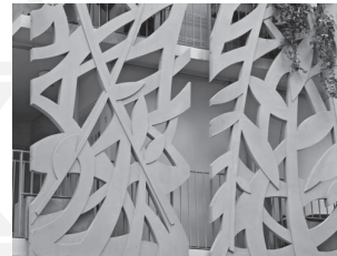
III. 13. Application of RPC (Reactive Powder Concrete) – “Ductal®”: cladding (façade) elements, a – Museum of the Civilisations of Europe and the Mediterranean (MuCEM), Marseille, France, 2013 [51], b – housing block, ZAC Paris Rive Gauche, Paris, France, 2007 [52]
