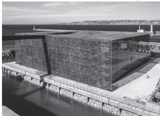
III. 13. Application of RPC (Reactive Powder Concrete) – “Ductal®”: cladding (façade) elements, a – Museum of the Civilisations of Europe and the Mediterranean (MuCEM), Marseille, France, 2013 [51], b – housing block, ZAC Paris Rive Gauche, Paris, France, 2007 [52]
