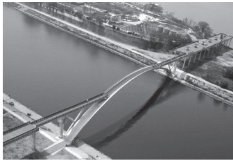
III. 6. Application of RPC (Reactive Powder Concrete) – “Ductal®”: “Seonyu footbridge” (“Footbridge of Peace”) – the longest footbridge in the world made of RPC (span: 120 m) (3 cm thick slab, \pi -shaped cross-section of the arch) – prestressed concrete structure, Seoul, South Korea, 2002 [24, 52]
