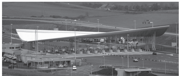
III. 8. Application of RPC (Reactive Powder Concrete) – “BSI/CERACEM®”: shed: Millau Viaduct Toll Gate, Millau, France, 2004 [49, 56]
