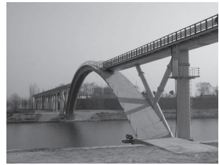
III. 6. Application of RPC (Reactive Powder Concrete) – “Ductal®”: “Seonyu footbridge” (“Footbridge of Peace”) – the longest footbridge in the world made of RPC (span: 120 m) (3 cm thick slab, \pi -shaped cross-section of the arch) – prestressed concrete structure, Seoul, South Korea, 2002 [24, 52]
