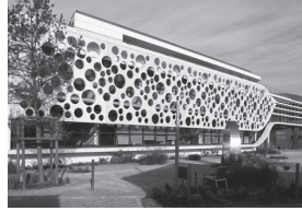
III. 12. Application of RPC (Reactive Powder Concrete) – “Ductal®”: façade panels – sun-shades (“double-skin façade”=“building envelope”), a – Plescop City Hall, Plescop, France, 2010, b – Rabat-Salé Airport building, Rabat, Morocco, 2011 [52]
