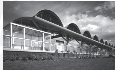
III. 7. Application of RPC (Reactive Powder Concrete) – “Ductal®”: Shawnessy Light Rail Train (LRT) Station (RPC precast elements: ultra-thin (2 cm) curved roof shell, columns), Calgary, Canada, 2004 [40]
