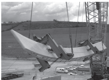
III. 8. Application of RPC (Reactive Powder Concrete) – “BSI/CERACEM®”: shed: Millau Viaduct Toll Gate, Millau, France, 2004 [49, 56]
