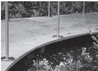
III. 14. Application of RPC (Reactive Powder Concrete) – “Ductal®”: pathway – “Flying Carpet”, Tomi Ungerer Museum – International Centre for Illustration, Strasbourg, France, 2007 [52]
