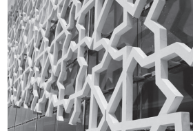
III. 12. Application of RPC (Reactive Powder Concrete) – “Ductal®”: façade panels – sun-shades (“double-skin façade”=“building envelope”), a – Plescop City Hall, Plescop, France, 2010, b – Rabat-Salé Airport building, Rabat, Morocco, 2011 [52]
