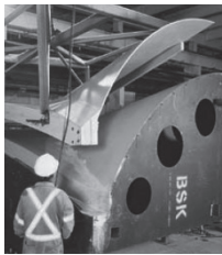
III. 7. Application of RPC (Reactive Powder Concrete) – “Ductal®”: Shawnessy Light Rail Train (LRT) Station (RPC precast elements: ultra-thin (2 cm) curved roof shell, columns), Calgary, Canada, 2004 [40]
