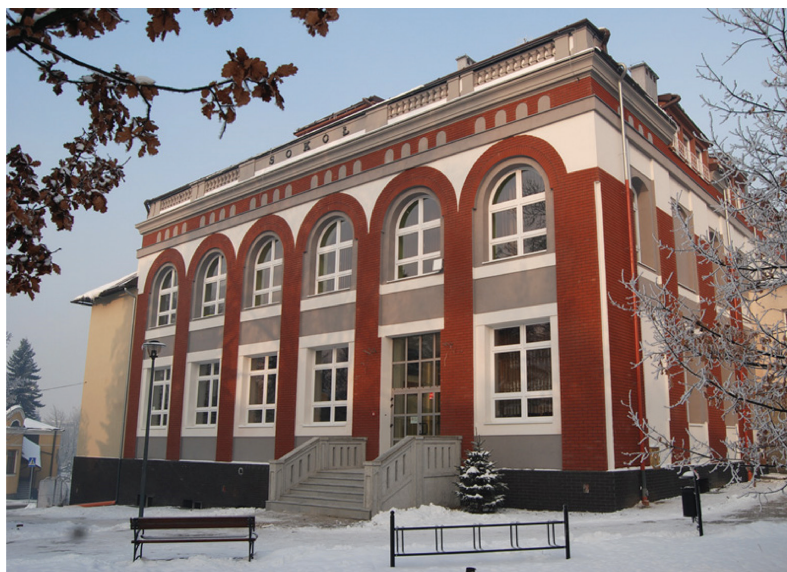
III. 1. Building of the former “Sokół” in Nowy Targ after thermomodernization (photo by D. Kuśnierz-Krupa, 2012, [in:] Archives of GP Zeriba)
