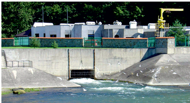
Fig. 4. A view of the hydroelectric power plant (Photo by B. Paluszkiewicz)
