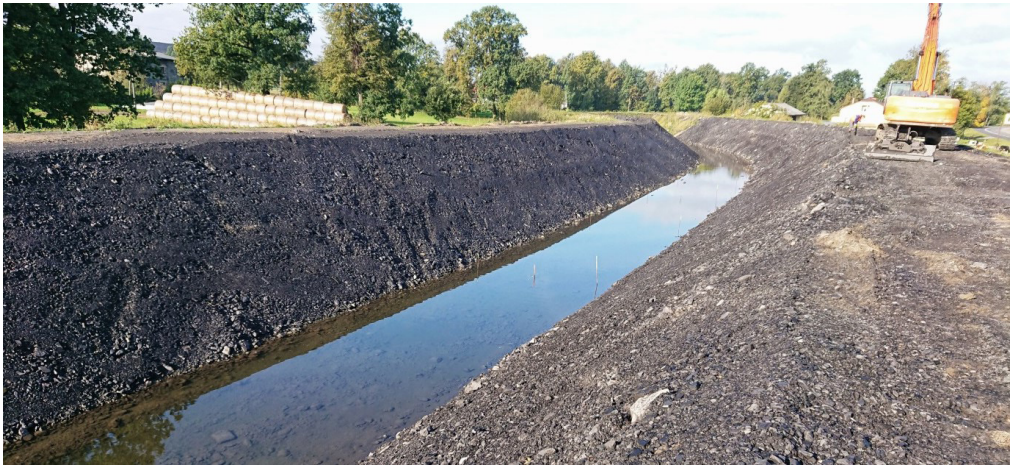
Fig. 7. Preparing riverbed for restoration
