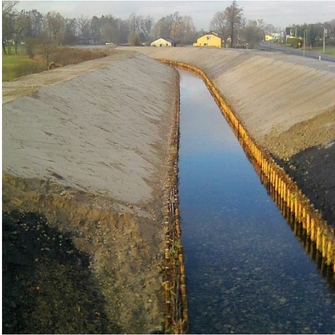
Fig. 8. Topsoiling of slopes
