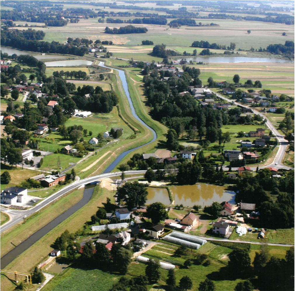
Fig. 10. Completed works after the most recent restoration
