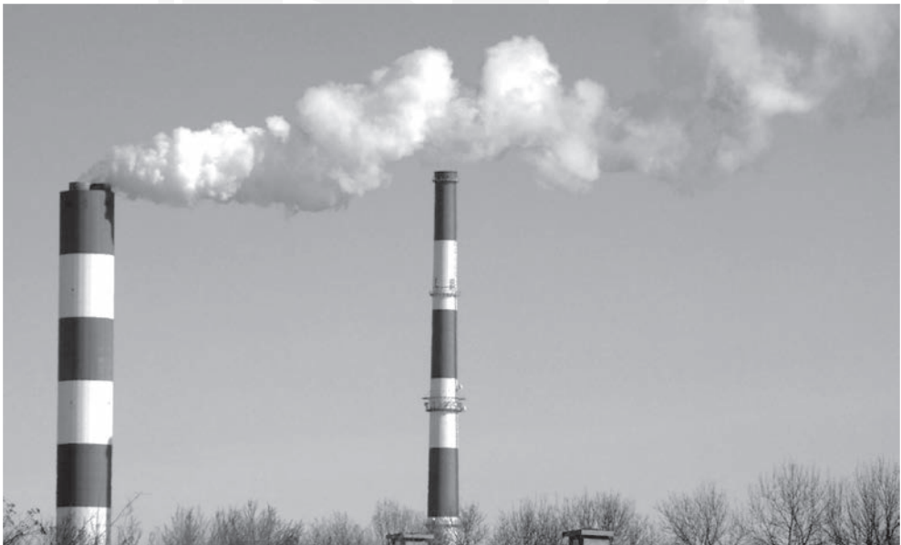
Fig. 1. Example of concrete structures exposed to environmental conditions
