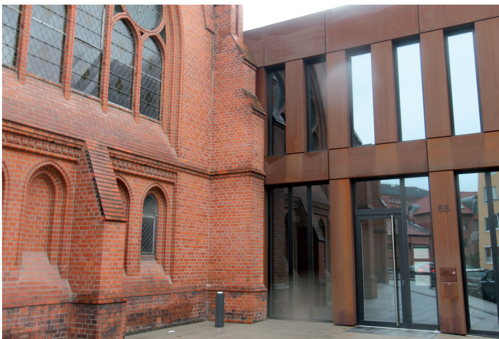
Ill. 11. Hannover, church of the Apostles, place of connecting the contemporary extension with the brick wall of the neo-Gothic church (photo by author)
