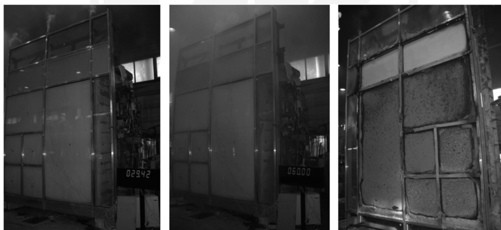
III. 2. The impact of fire on the curtain wall, visible movement of hot air and gases inside the carrier profiles (source: B. Sędlak, Fire resistance tests of glass curtain walls , part 2, in Świat Szkła (The World of Glass) 10/2012)
