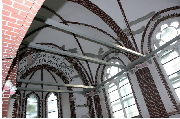
Fig. 5. Vault reinforcement set up for the duration of rectification
