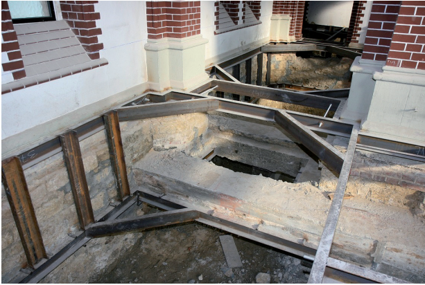
Fig. 4. Flooring reinforcement set up for the duration of rectification
