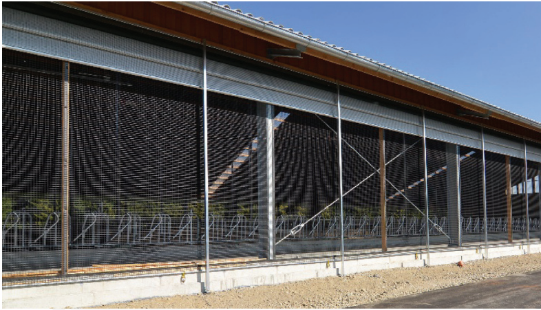
Fig. 1. A utility building with openwork side walls
