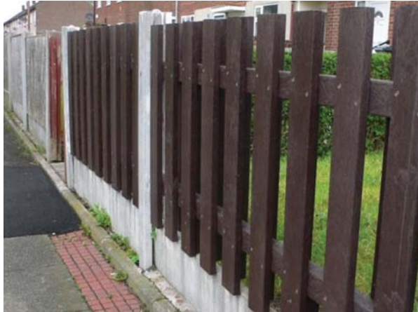
Fig. 8. Example of fence made of waste polystyrene [16]
