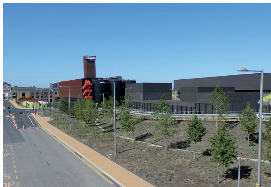
III. 4. The Copper Box, multifunctional sport arena located in the Olympic Park in London, designed by the Make Architects (photo by author)
