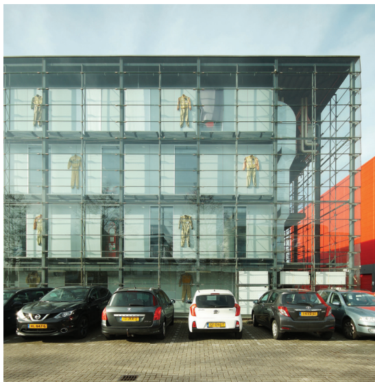
Fig. 11. Go-cart racing track in Delft (arch. Cepezed, 2001)
