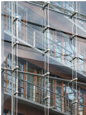
Fig. 25. H 19 Office Building in Duesselfor (arch. Petzinka Pink und Partner, 2002)
