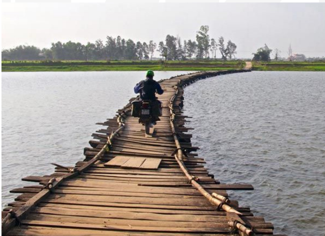
Fig. 18. An example of a contemporary “modern” wooden bridge in Vietnam (source: https://s-media-cache-ak0.pinimg.com/736x/ae/90/cd/ae90cddc187a70b5421b82814553f14e.jpg , access: April, 2016)
