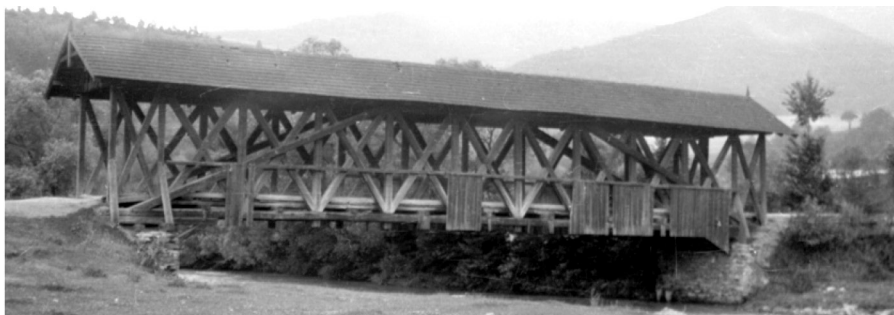
Fig. 10. Combined system of covered timber truss bridge used in Kluknava (Courtesy of The Monument Boards of The Slovak Republic)
