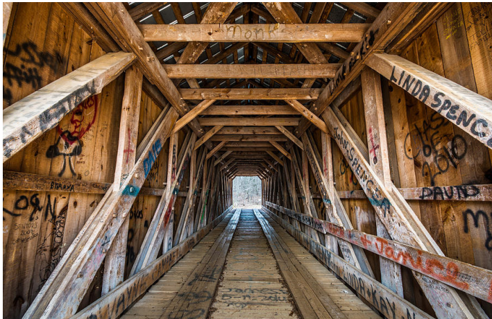
Fig. 16. Entrance to the Bunker Hill Covered Bridge (source: http://images.fineartamerica.com/images-medium-large-5/bunker-hill-covered-bridge-2-randy-scherkenbach.jpg , access: April, 2016)
