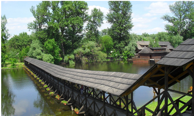
Fig. 17. The covered timber bridge in Slovak Kolárovo – the longest bridge in Europe built entirely of wood (source: https://upload.wikimedia.org/wikipedia/commons/thumb/1/14/G%C3%BAta093.JPG/1280px-G%C3%BAta093.JPG , access: April, 2016)
