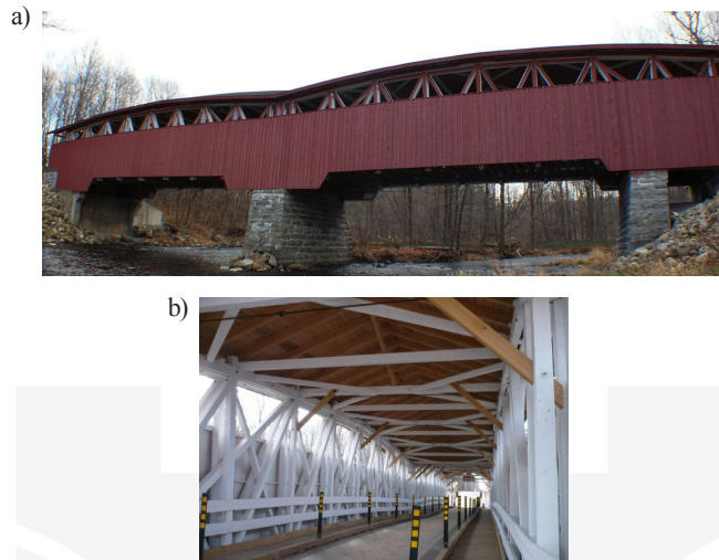
Fig. 11. The Percy Covered Bridge built in Powerscourt in the Province of Quebec – the oldest heritage timber bridge in Canada which remains in service (sources: a) https://c1.staticflickr.com/1/646/23671000872_e29a8ee27a_b.jpg , access: April, 2016, b) http://static.panoramio.com/photos/large/34017925.jpg , access: April, 2016)
