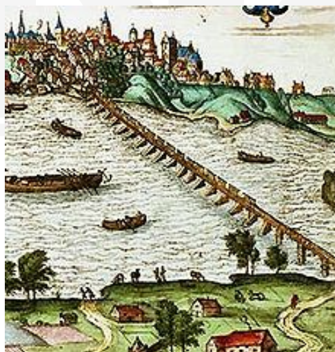
Fig. 6. The Sigismundus Augustus timber bridge over the Vistula River in Warsaw in the old picture (source: https://upload.wikimedia.org/wikipedia/commons/0/0a/Sigismundus_Augustus_Bridge_in_Warsaw.jpg , access: April, 2016)
