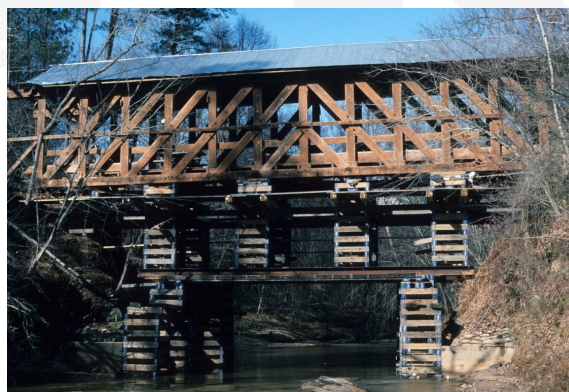
Fig. 15. The heritage Bunker Hill Covered Bridge in North Carolina in the USA with the Haupt's type wooden truss girder (source: http://d.lib.ncsu.edu/collections/catalog/bh0241pnc006 , access: April, 2016)
