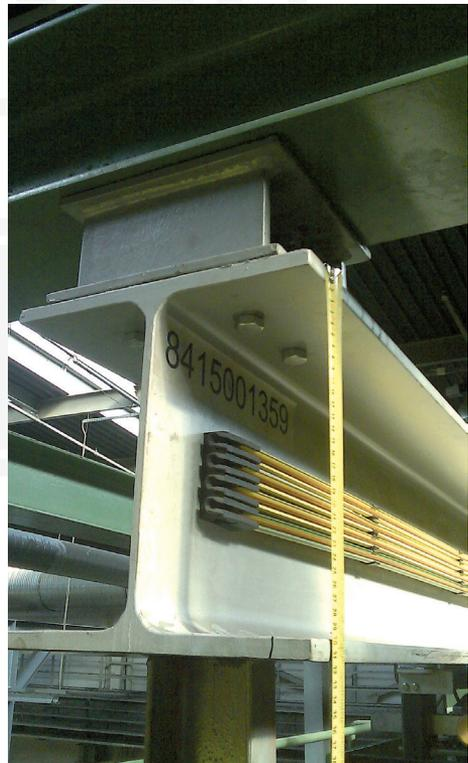
Fig. 8. Front view of the box bracket (connected to 4M 8.8), securing the load-carrying beam of the travel track (photo. from the author's archive)
