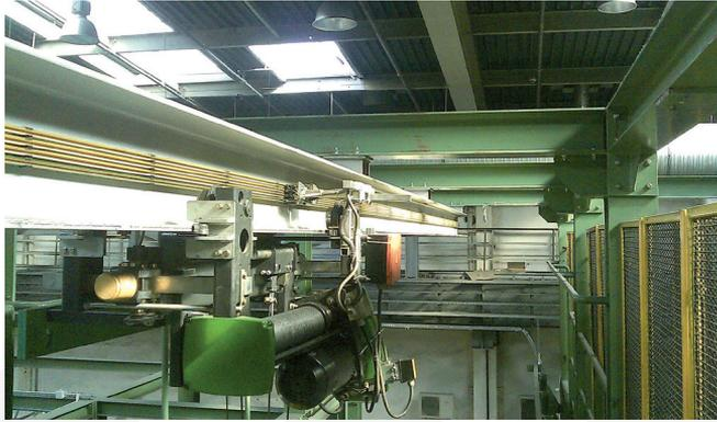
Fig. 6. View of the technical crane. The lower flange of the wide-flange HEA 320 beam constitutes the travel track (photo. from the author's archive)
