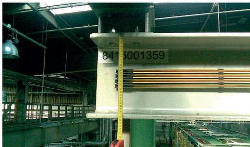
Fig. 9. Free end of the track beam together with the box bracket, fastened to the framework system. Study of the load-carrying system (photo. from the author’s archive)
