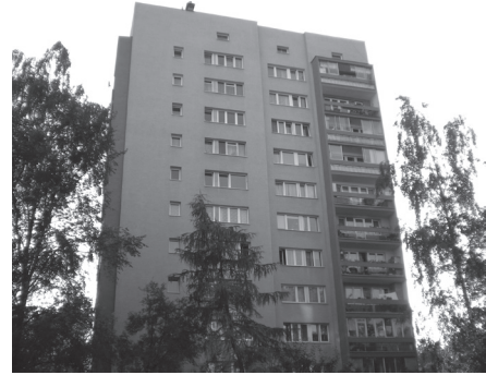
III. 2b. Building #2 – East elevation
