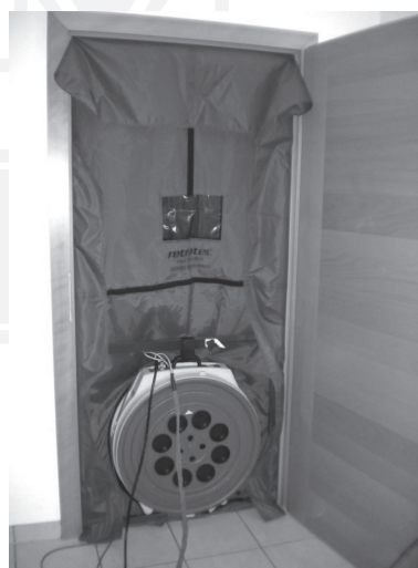
Ill. 1b. Blowerdoor set the in the Flat number 2
