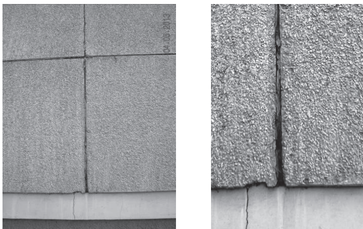
III. 5. System joint in building number 1 – external view
