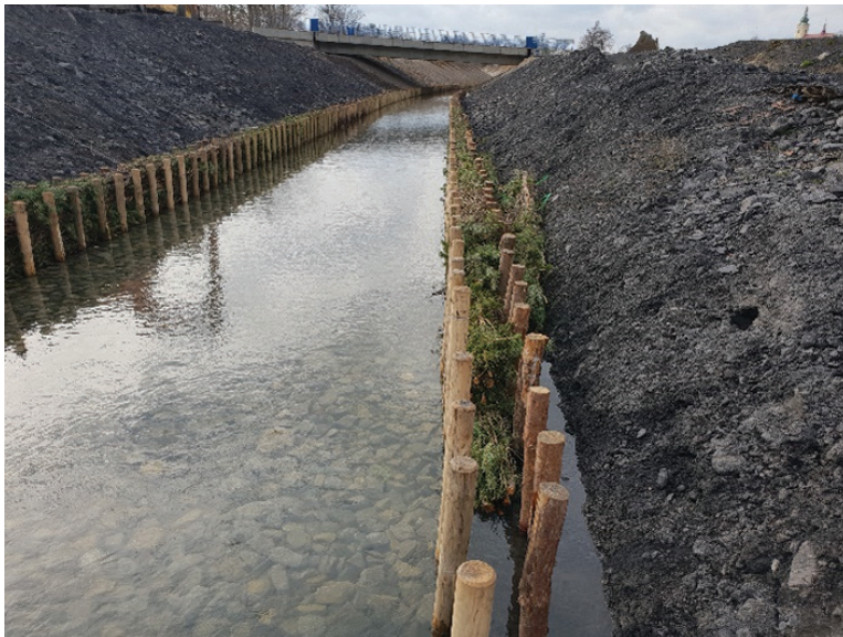
Fig. 10. Works related to the incorporation of fascines and humus – covering the scarps along the Pszczyńska river
