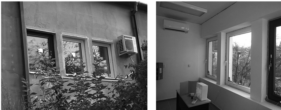
Fig. 1. Exterior and interior of climatic chamber with integrated samples of window constructions
