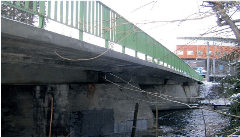
Fig. 1. The analysed bridge in Wisla (photo by authors)
